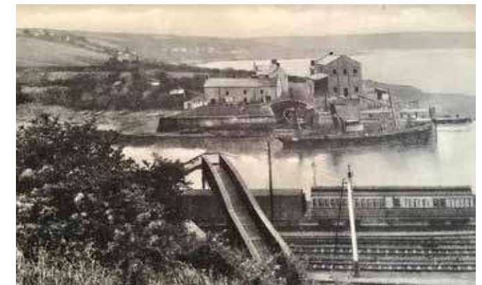
The footbridge - with Ice Factory in back ground.
